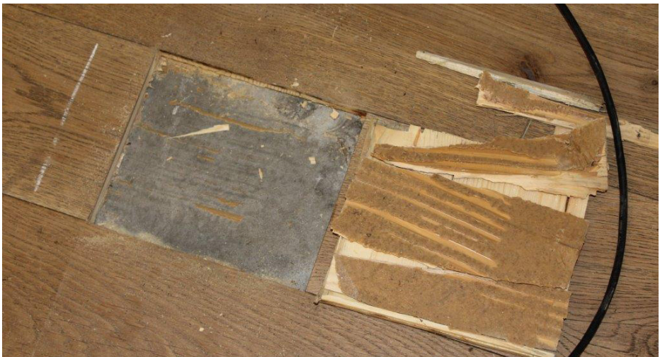
Detached parquet on screed
