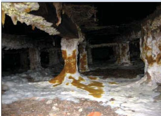
Fig. 1: Genuine dry rot infestation of a balcony substructure
